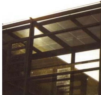
Amorphous silicon can be made into semitransparent modules.
